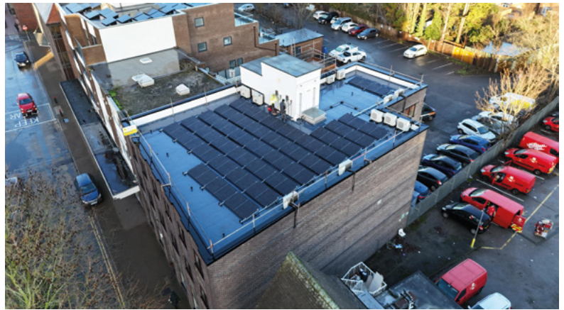
Solar panels are expected to meet around 25% of the building's annual electrical demand
